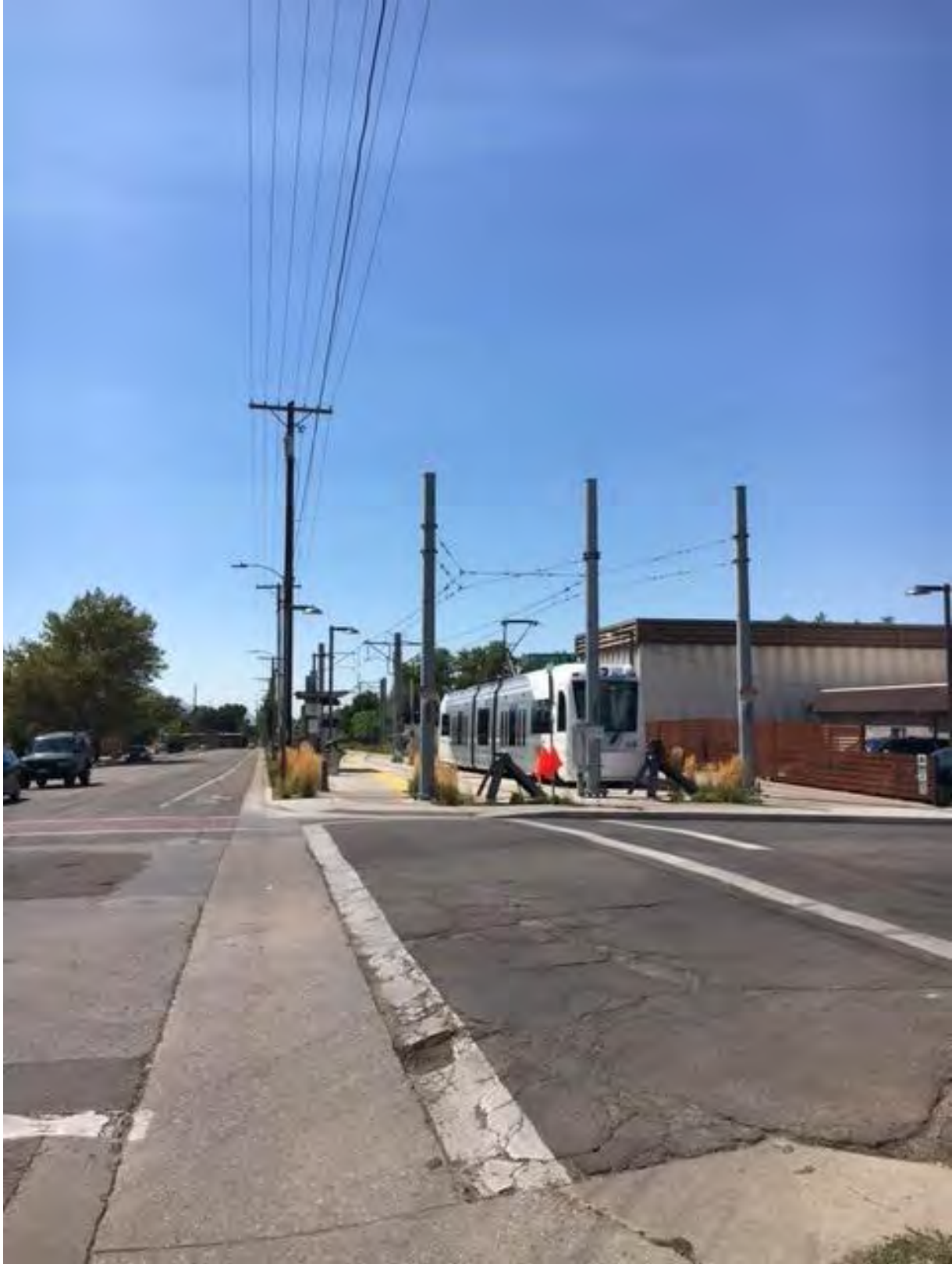
Looking towards the west along Sugarmont Drive. The S-Line Fairmont stop can be seen at the right.
