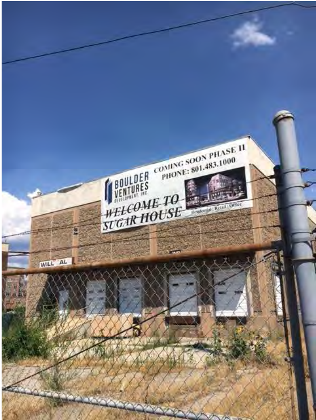
This photograph is looking towards the northeast at the existing warehouse on the site.
