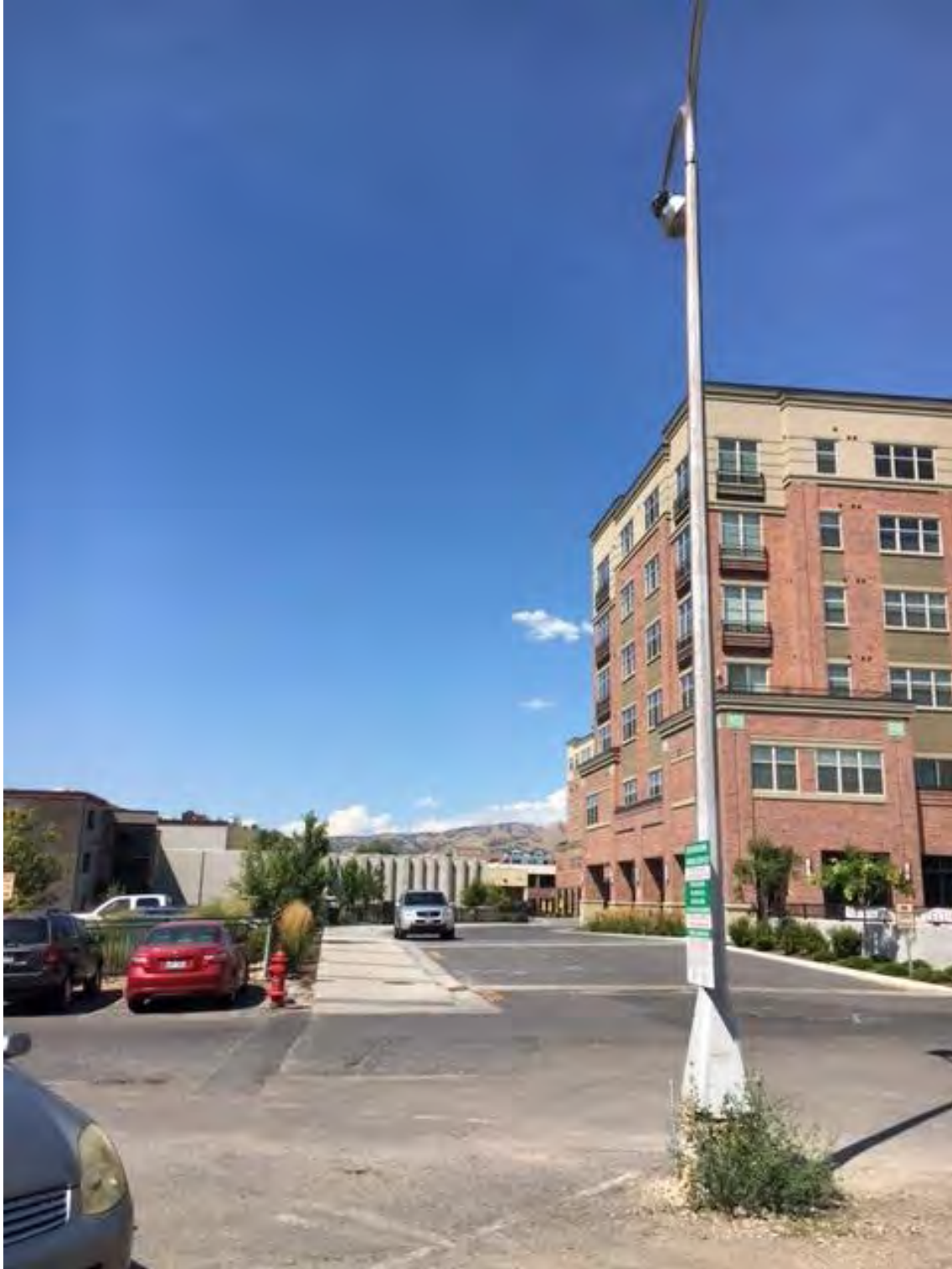
This photograph is looking towards the north in the center of the Granite Block. The Vue Mixed-Use project is on the right and the pedestrian walkway connecting to 2100 South is in the center of the photograph.
