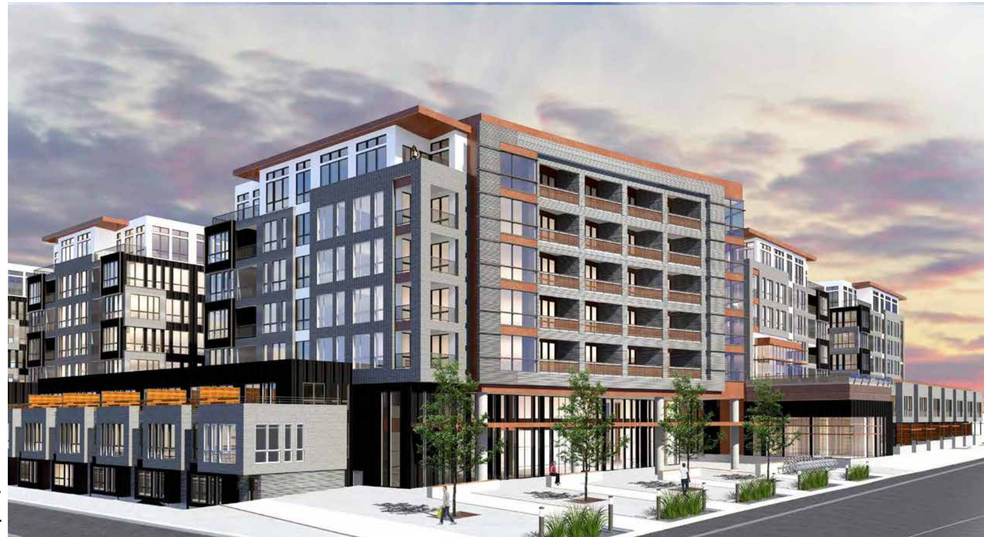
VIEW LOOKING NORTHEAST FROM CORNER OF McCLELLAND AND SUGARMONT
